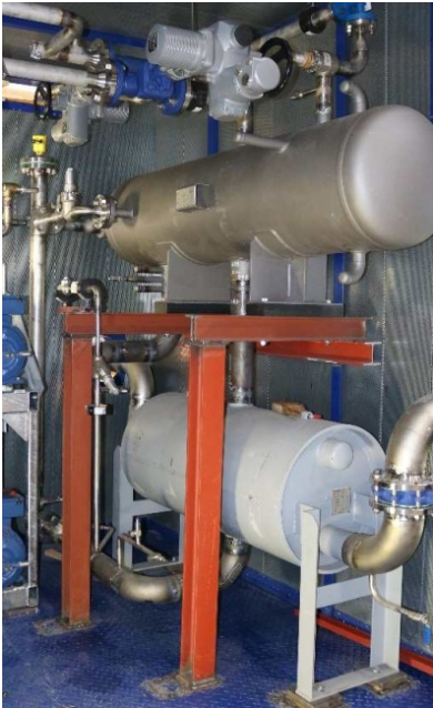
Flooded CO 2 evaporator with separator Type: XPS 50 Design: Fully welded Special features: design pressure 120 bar Installation site: mobile in a container
